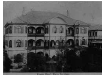
141 Kyoto Hotel, Main Bldg.
