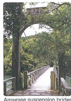
Amagase suspension bridge
